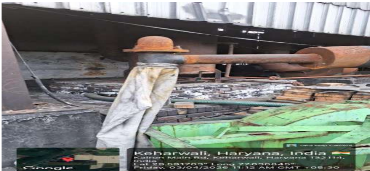
2.4.7 Photograph of suction hood attached to a bag filter
